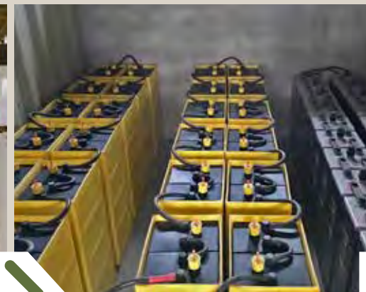
That energy is converted into energy stored in battery banks
