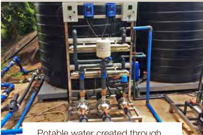
Potable water created through a reverse osmosis plant
