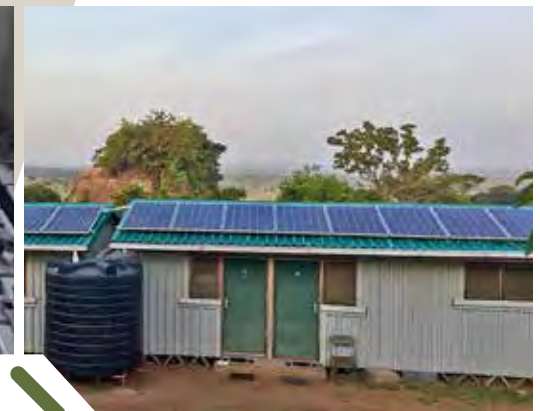
And all systems controlled remotely from an off site office
