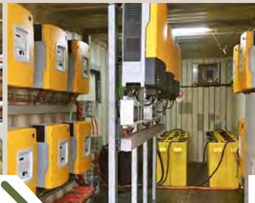
Supply energy to inverters
